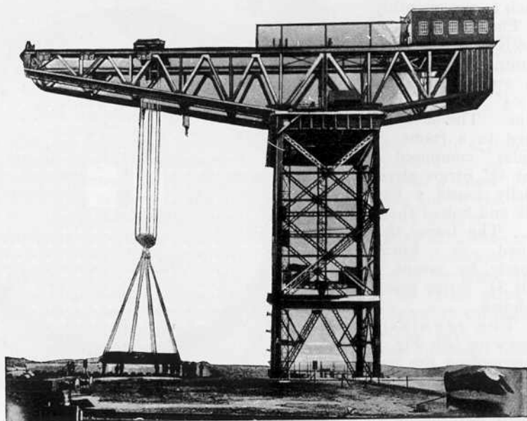
Fig. 2. A Giant Hammerhead Crane at work.
